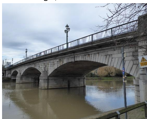
Staines Bridge constructed in 1832
